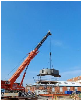
Finalise hull build APCL Falmouth
