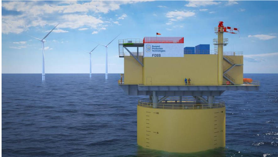
Floating substation technology for FLOW projects
