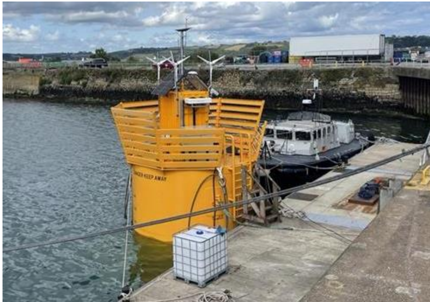
Photo of platform in the water demonstrating the in-water profile.
